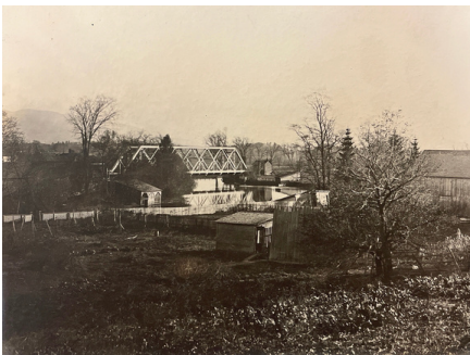
Railroad Bridge, Middlebury, VT Porter Collection
